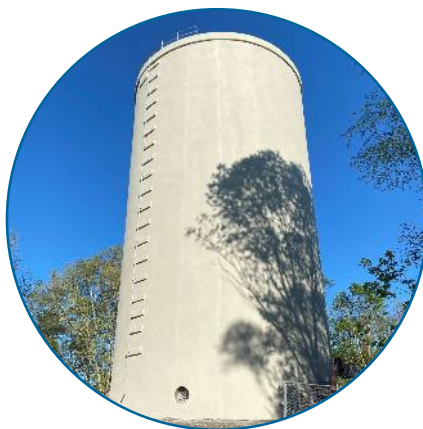
Patty Lane Tank Plainfield
